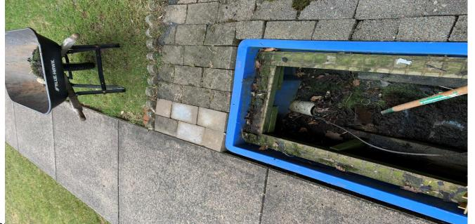
Several wheelbarrow loads of sediment were removed from the catch basin. The pavers were leveled, and weeds were removed. This will prevent the drainage system from clogging and will keep surface water flowing away from the building.
